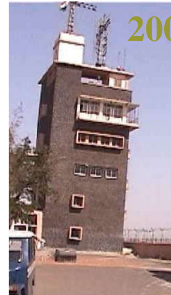
Kandla port building after 2001 Bhuj earthquake
