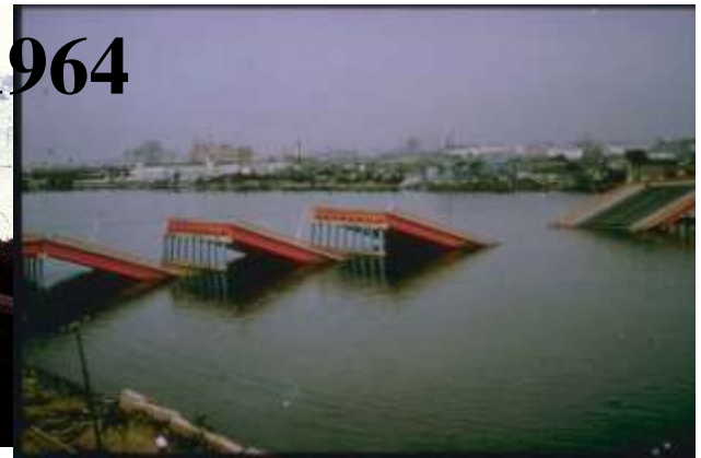
Showa Bridge after 1964 Niigata earthquake
